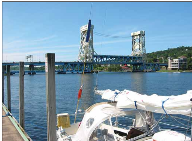
Portage Lake Lift Bridge connects Houghton and Hancock, Michigan.
