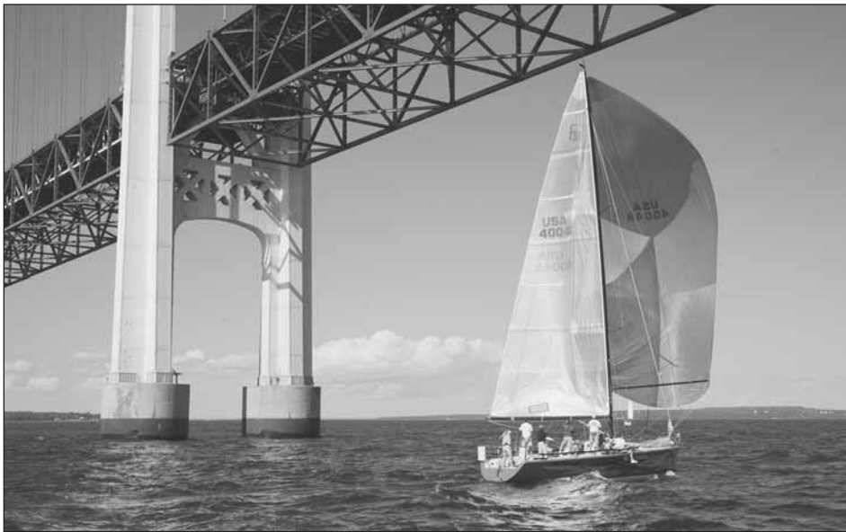
Inferno blazes it's way under Mackinac Bridge. Photo provided by Boatingshots.com.
