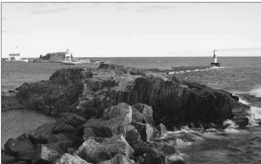
Grand Marais Harbor Breakwater, Lake Superior, North Shore of Minnesota.
