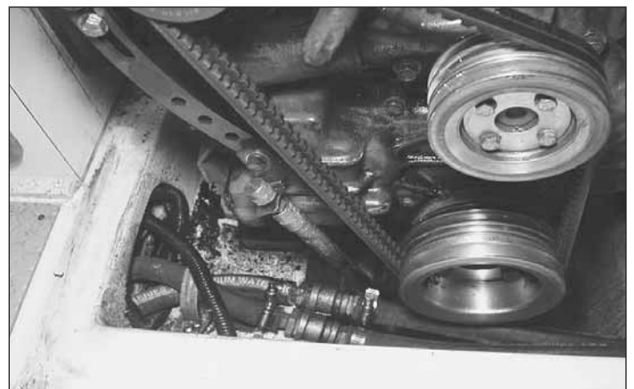
Still a mess even after cleaning up and new belts.
